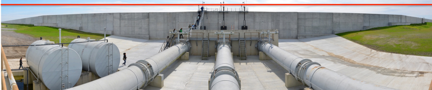
Figure 1: “The Great Wall of Louisiana,” Hurricane & Storm Damage Risk Reduction System (HSDRSS), St. Bernard Parish, Louisiana, US Army Corps of Engineers (photo credit: Derek Hoeflerlin, 2012).
